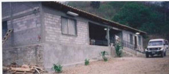
Santa Lucia Clinic Construction
